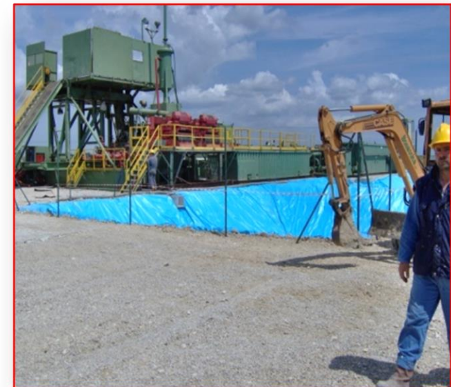
Waste management area
